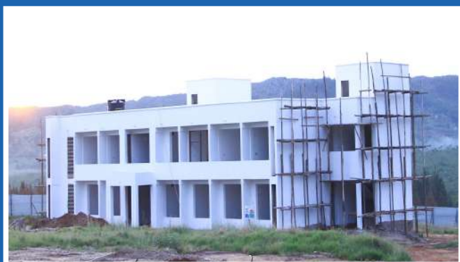
Assured Accommodation: A new hostel building, constructed under HEET project, at UDSM Kagera campus.
